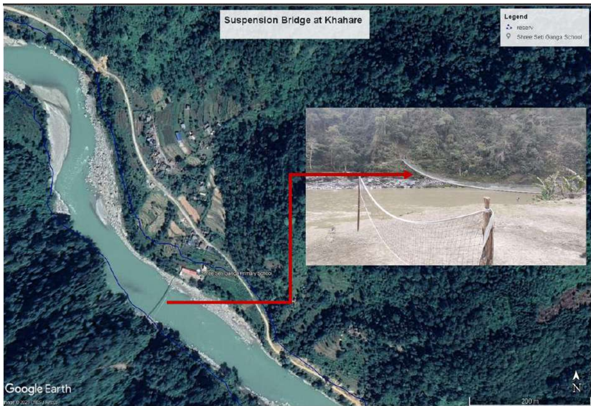
Figure 100: Suspension Bridge at Khahare, bandipur-6
