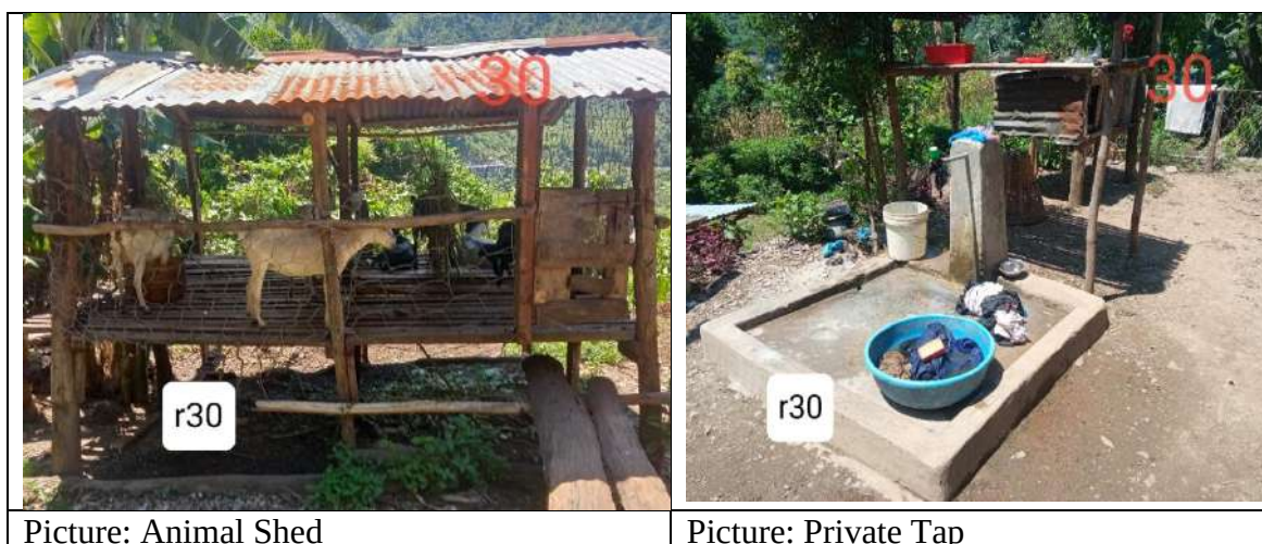
Figure 94: Some of the affected structures
